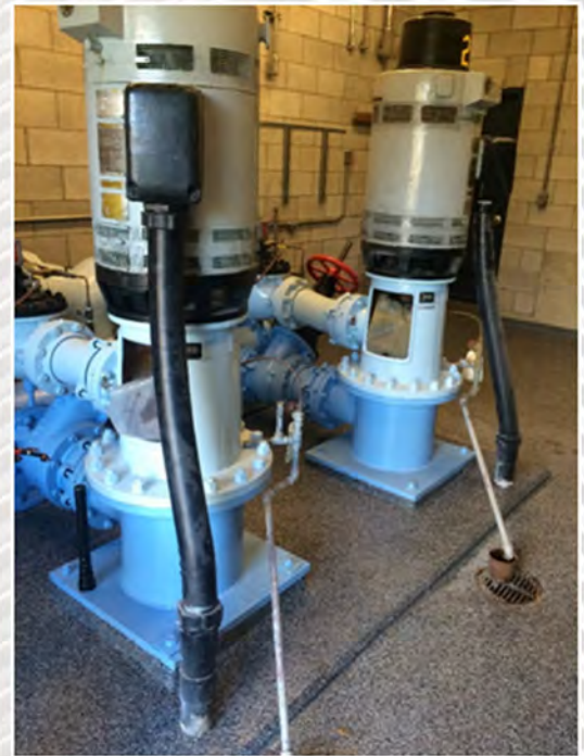
Vertical turbine pump
